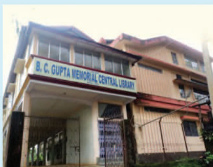
Central Library Building
